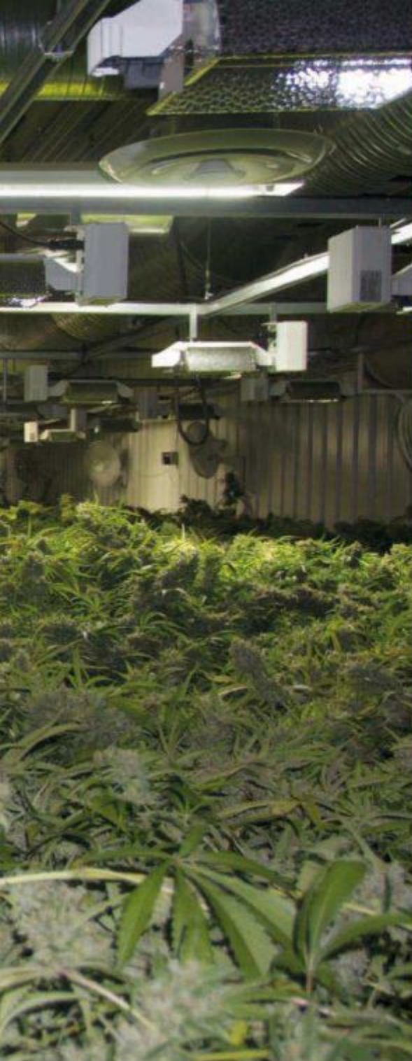
The vegetation area is lit with LEP (light-emitting plasma) and MH (metal halide) lighting. Right: A laboratory provides tissue culture specimens.
